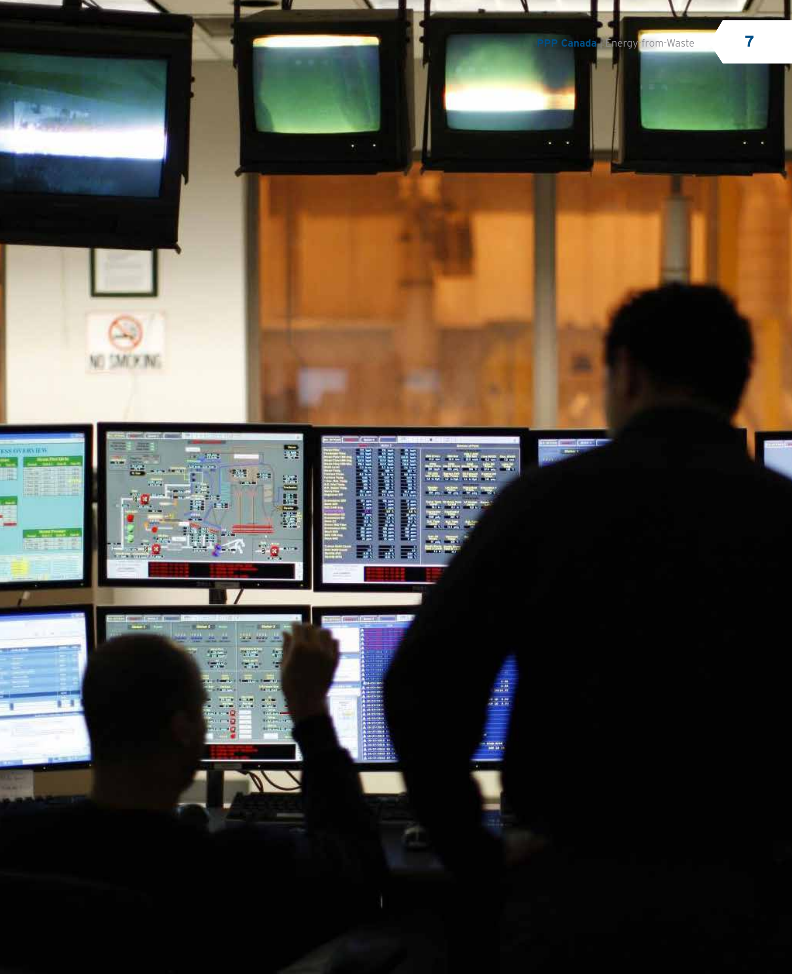
Photo Courtesy of: Covanta Indianapolis Energy-from-Waste facility, Mass Burn; in operations .
